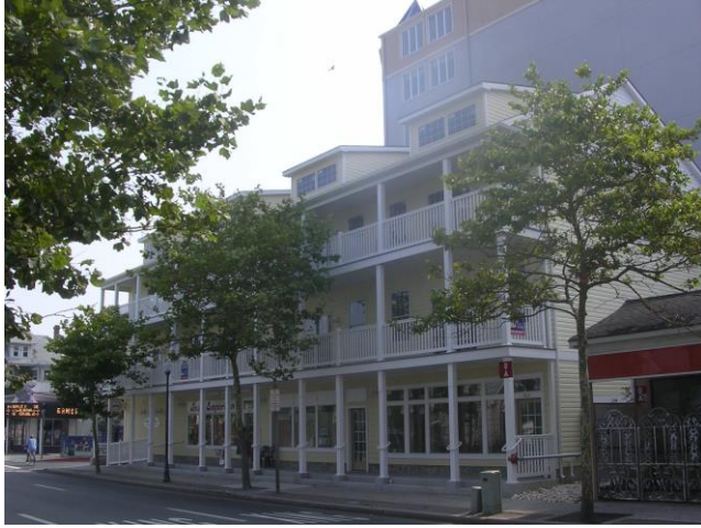
Boards Edge Villas mixed use project located at Baltimore Avenue and Talbot Street.
