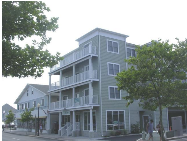
Elliott's On the Avenue mixed use project on Baltimore Avenue north of Wicomico Street.
