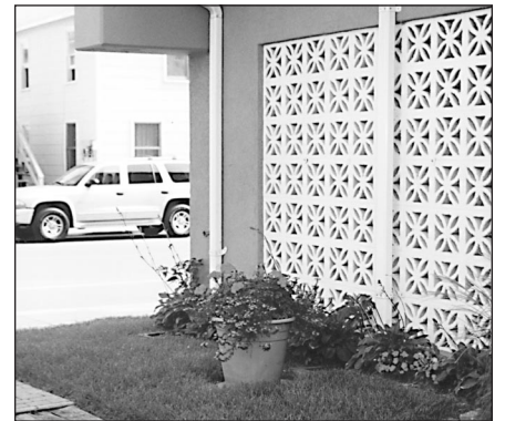
Screening of first floor parking area.
