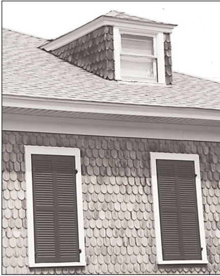
Walker House Baltimore Avenue - 1910
