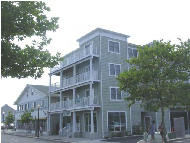
Elliott's On The Avenue mixed use project on Baltimore Avenue north of Wicomico Street.
