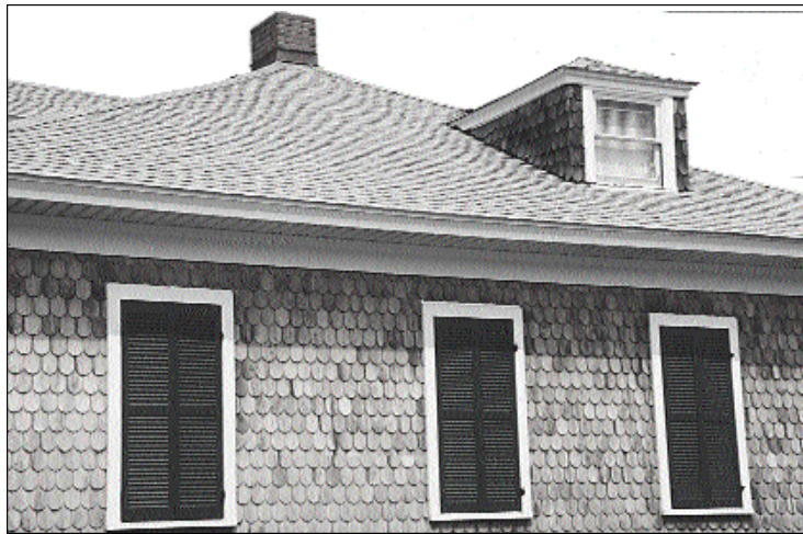
Walker House Baltimore Avenue 1910
