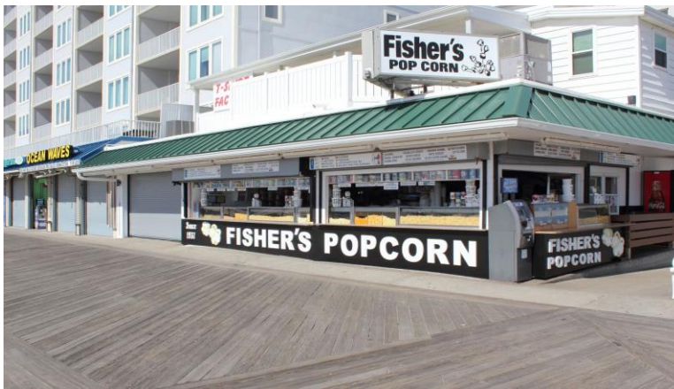
After (new raised awning and screening of mechanical equipment) 200 S. Atlantic Avenue – commercial property
