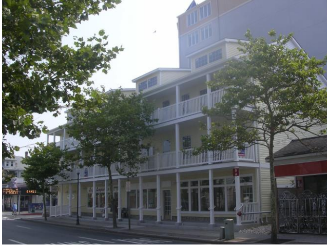
Boards Edge Villas mixed use project located at Baltimore Avenue and Talbot Street.
