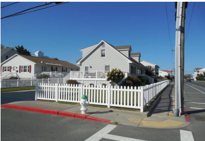
A new fence was completed under the OCDC Fence Streetside Program at 1101 St. Louis Avenue.
